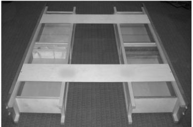
Attach 2 of the plywood deck pieces across the top near either end of the storage rails (See image above) using a #10 x 1 ½" screw in the hole at the end of each piece. The remaining holes will not be utilized.
