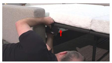
Install 2 Bolts through the Bracket on each side
