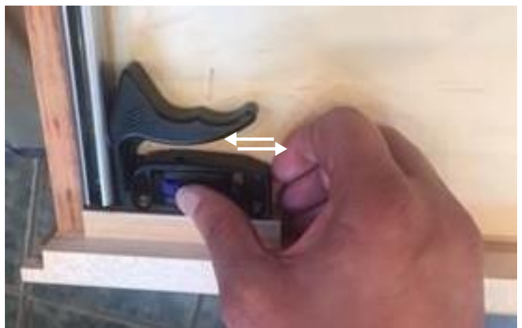
Figure 3. Level the drawer slides
