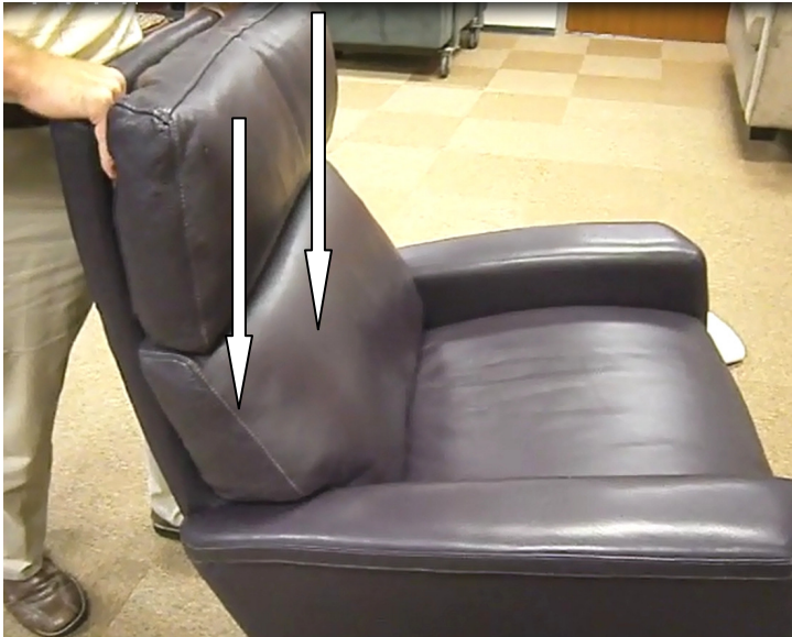
10. Push the Back upright and press down hard on the top of the Back to set the Spring Clips.
